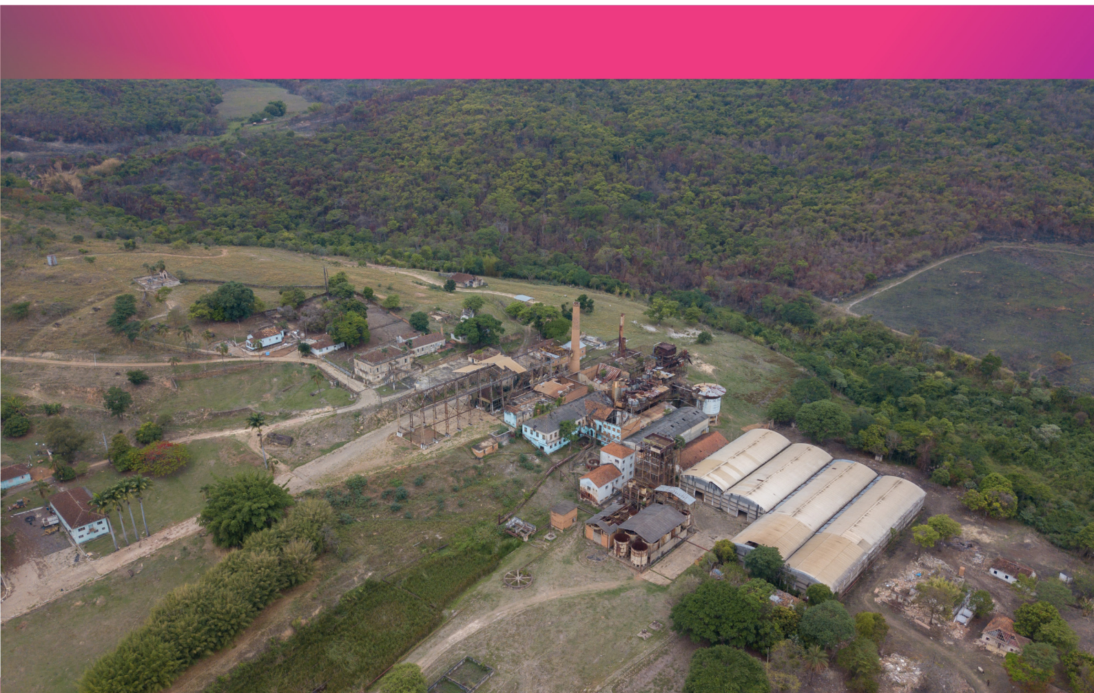
Aerial photo of ruins of the plant that originated the MST occupation in Campo do Meio (MG)
