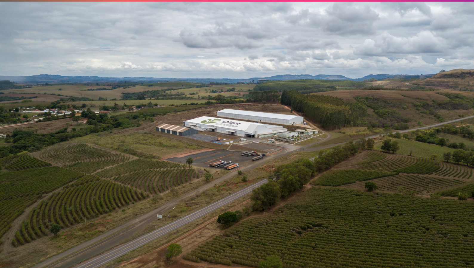
OLAM facilities at São Sebastião do Paraíso, MG
